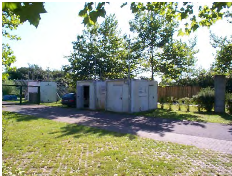
Figure 19: Field test site „Cologne, parking lot“
