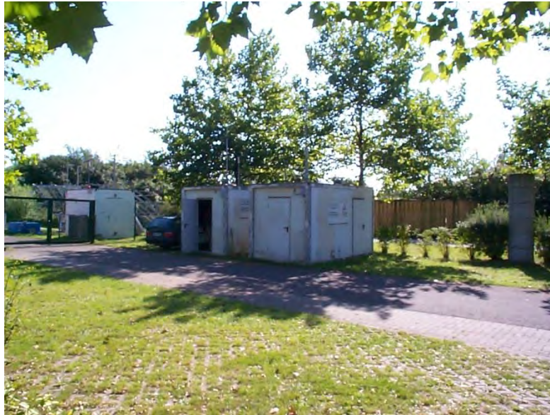
Figure 25: Field test site Cologne, parking lot
